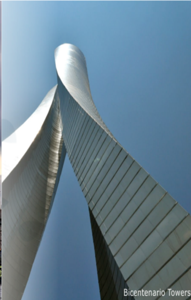
Bicentenario Towers 170m Toluca, Mexico
